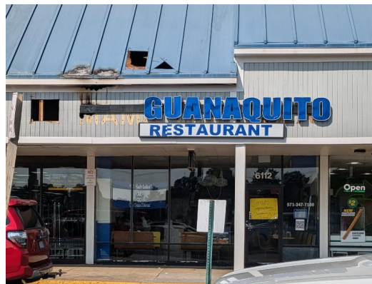
Fire damaged the sign for El Guanaquito restaurant. (Photo: Daniel Bearth)
