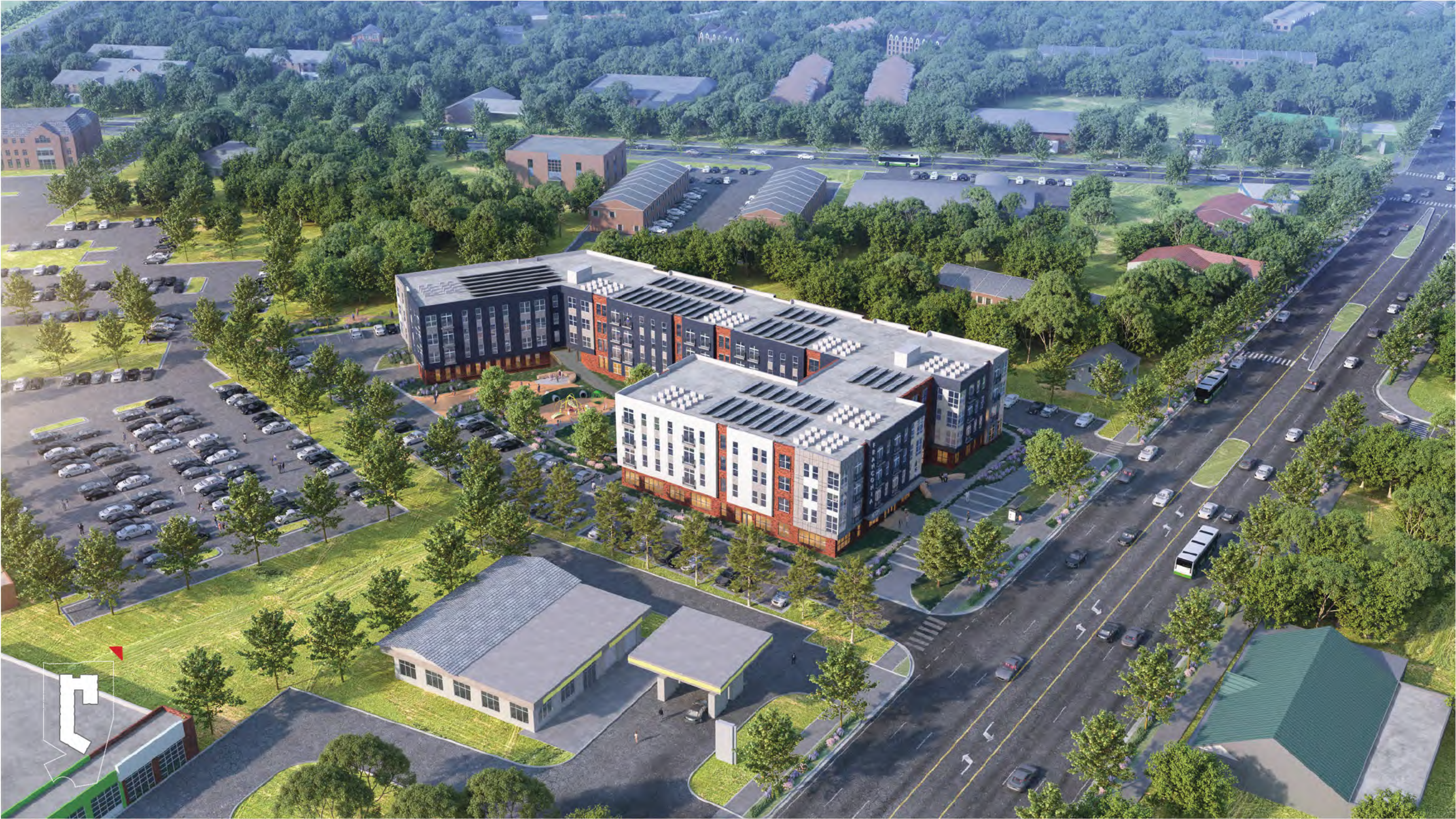
AERIAL VIEW TO SOUTHWEST
