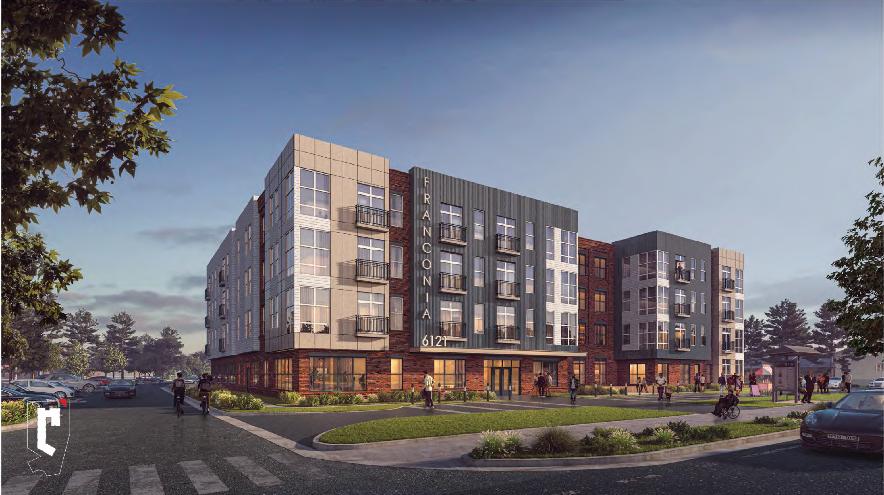
VIEW OF MAIN FACADE AND MAIN ENTRY
